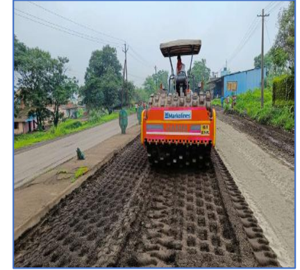
Compaction by Pad Foot Roller
