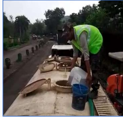
Addition of Liquid Chemical Additive
