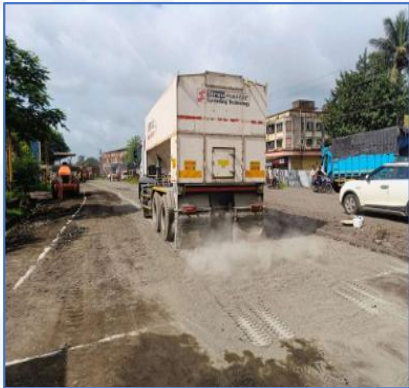
Cement Spreading by Microprocessor Controlled Spreader Truck
