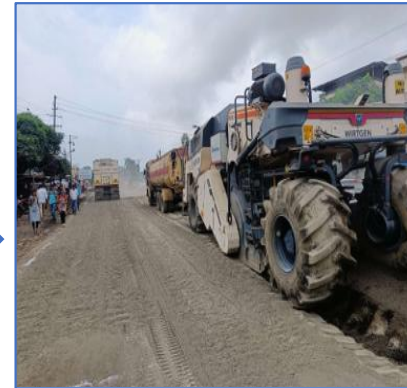
Pulverization of soil with Recycler
