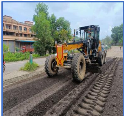
Grading & Profiling with motor Grader
