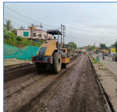
Compaction by Soil Compactor
